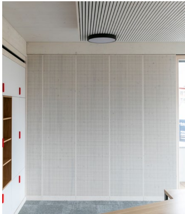
Drilled profile with surface treatment
